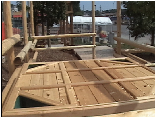
Nature Art table under construction
